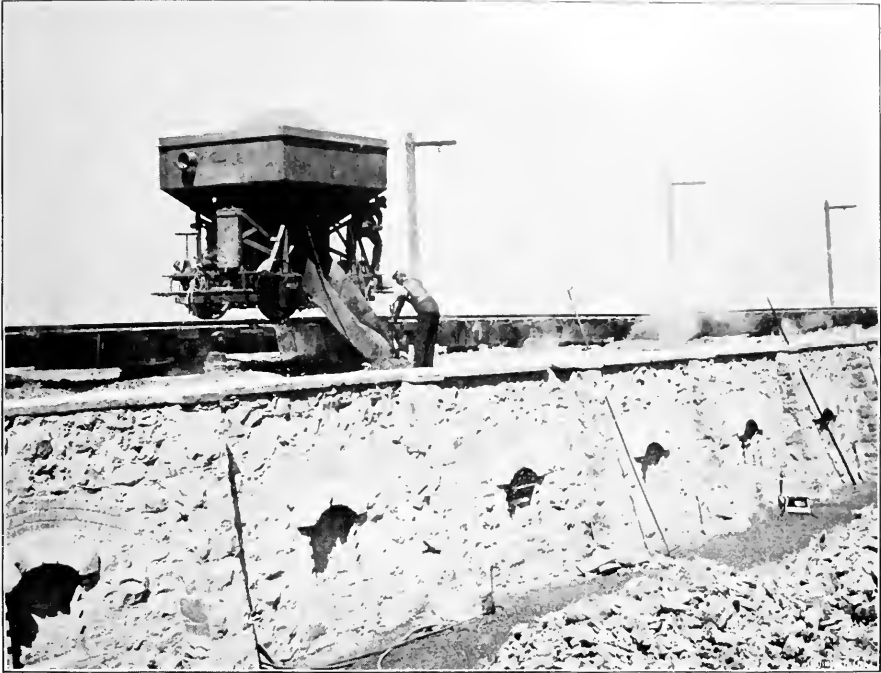
ELECTRIC TROLLEY—CHARGING COKE OVENS—FERNIE.
